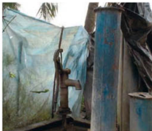
Defunct. Numerous arsenic-removal units installed by the West Bengal government no longer work due to lack of maintenance.
